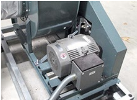
Air conditioner intake/exhaust fan upgrades (Energy saving)
