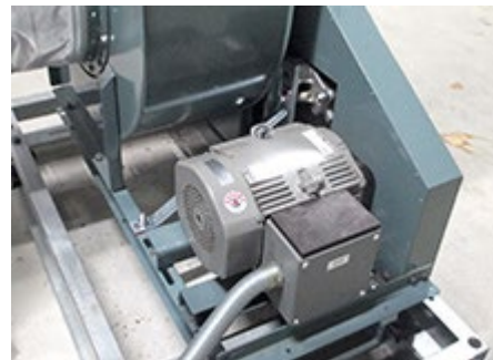
Air conditioner intake/exhaust fan upgrades (Energy saving)
